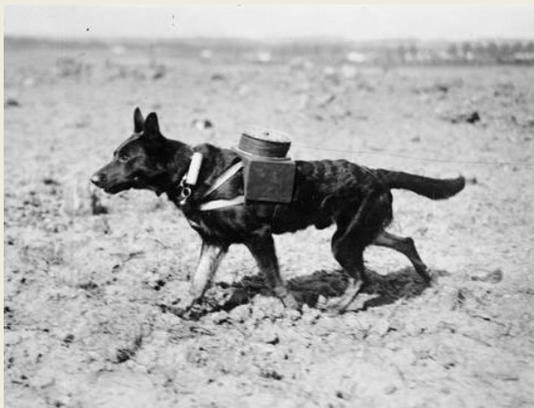
Lay telephone cables
